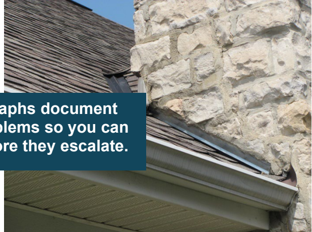
Flashing detail at chimney
